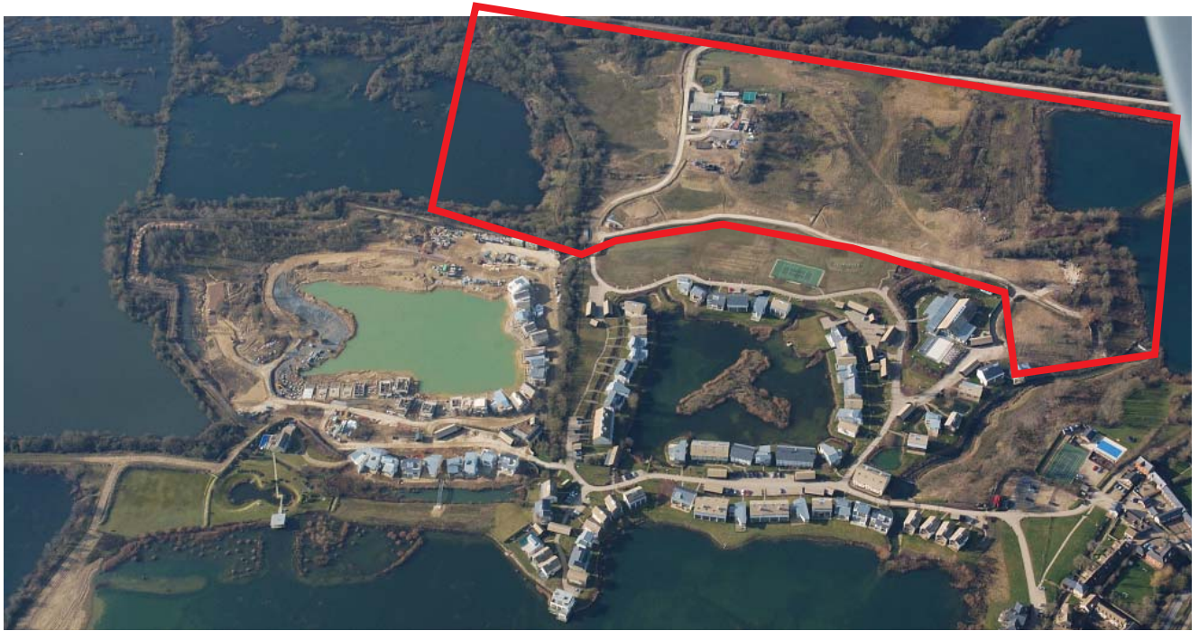
Lower Mill Estate Development
